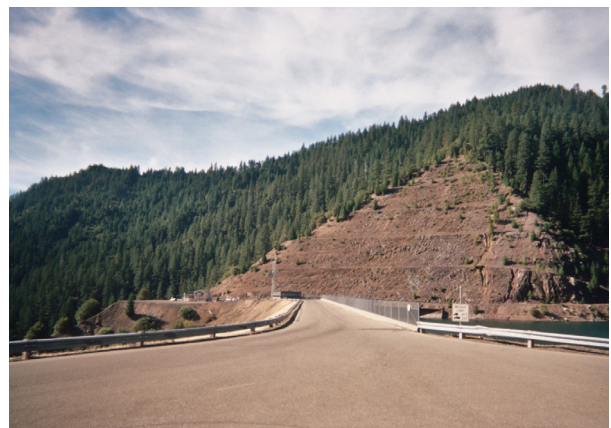
Road across dam
